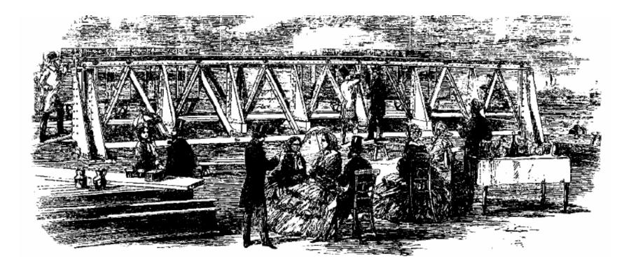
Testing of a steel truss in England for a railway bridge in India in the 19th century
